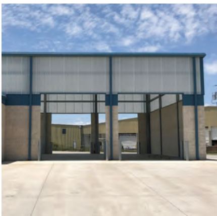
CMU block exterior with translucent paneling on the top to allow light in.
