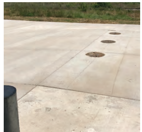
Sand/Mud Interceptor tanks allow time for separation of the solids from the water.
