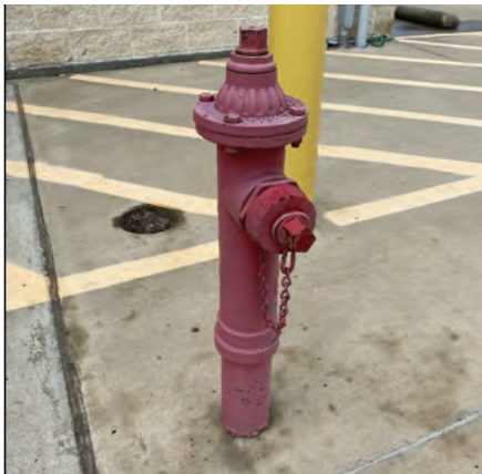
Exterior hydrant with 2.5" NST connection for fire hose. Full draining capability to prevent freezing.
